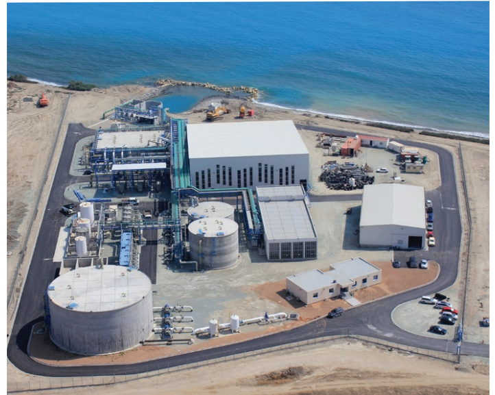
Courtesy of MN Limassol Water Co Air view photograph of Limassol Desalination plant.
